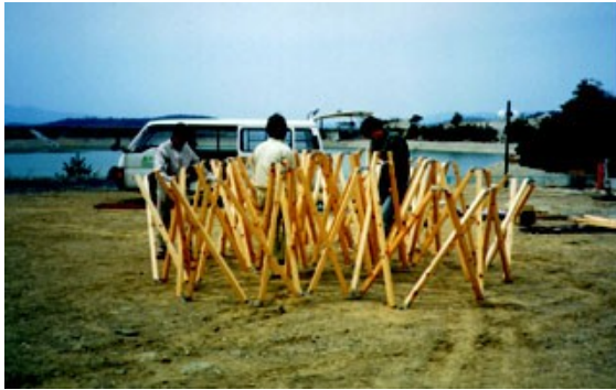
Hamanizuki Park deployable dome
